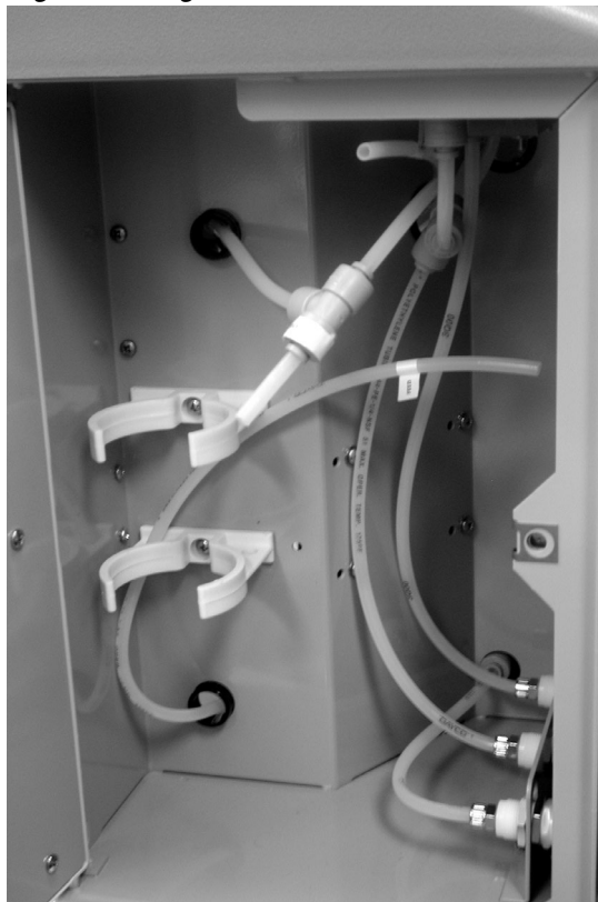
Figure 7 Single Membrane Installation
