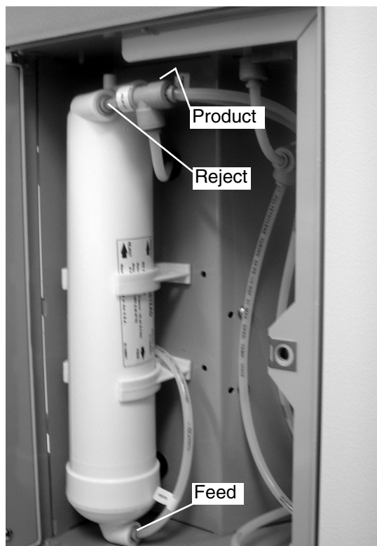
Figure 8 Single Membrane Installation
