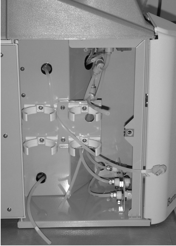
Figure 10 Double Membrane Installation
