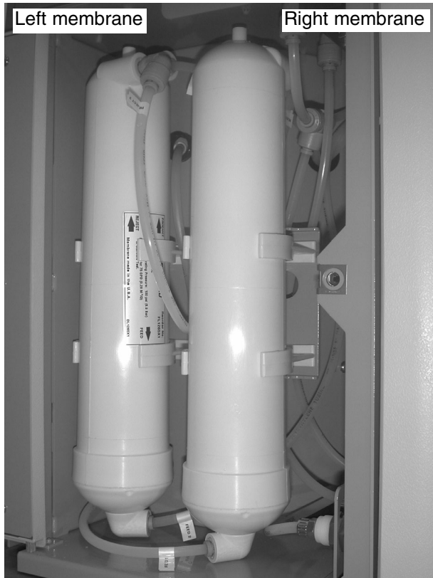
Figure 12 Double Membrane Installation
